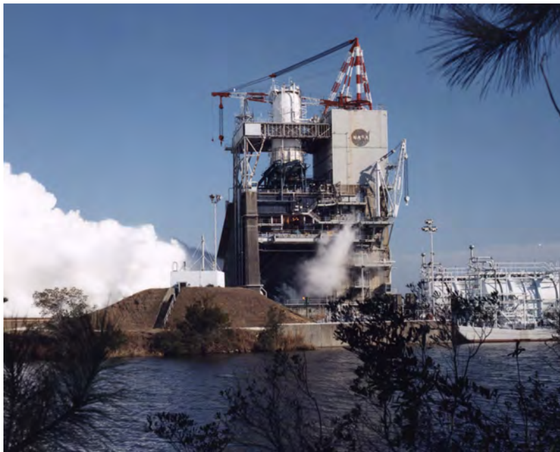
Rocket engine test stand at Stennis Space Center
